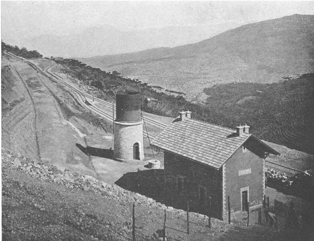
The reversing spur at Chouit-Araiya, 16km from Beirut and 550m (1,830 ft) up, seen in the 1950s. The track climbs at top left after arriving from below just to the right of that.
